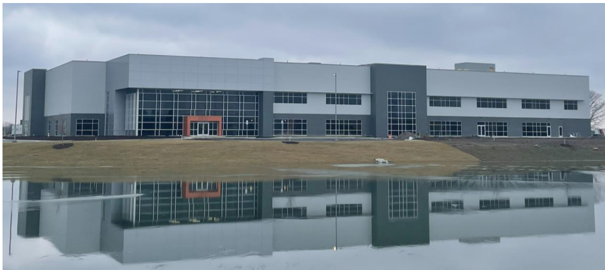
INCOG BioPharma Services ~90,000 square foot manufacturing facility and global headquarters, located in Fishers, IN.
